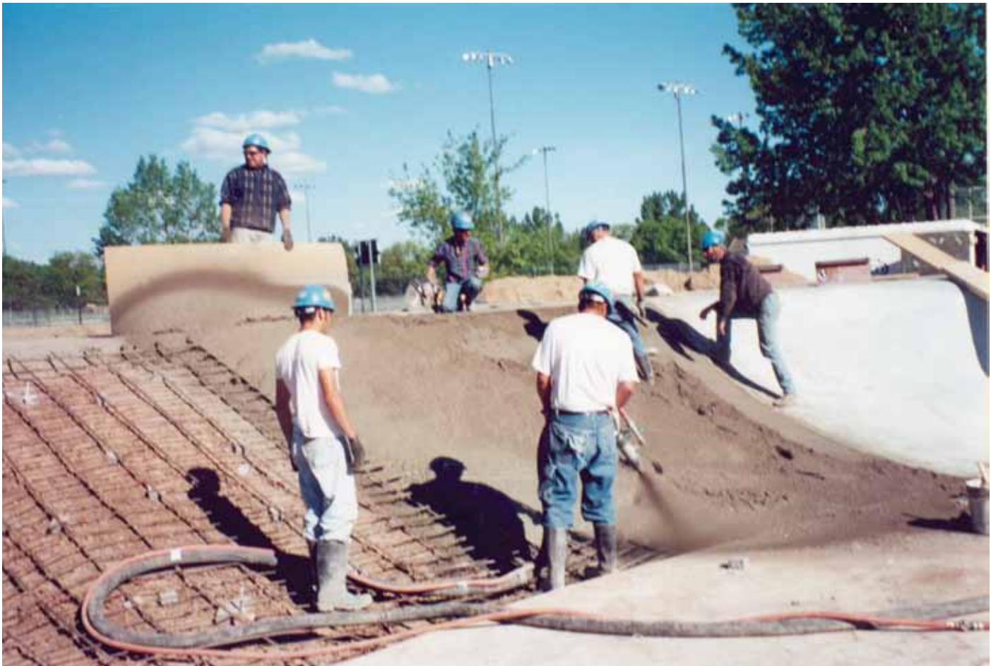
Shotcreting (wet gunning) with a stiff, low-slump shotcrete mix is all in a day's work for the Mayco C30HD.
