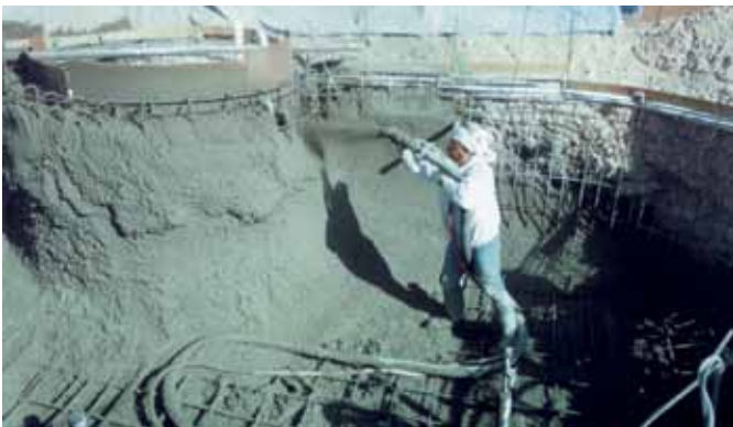
The LS500, with its powerful ability to handle the toughest shotcrete mixes, enables a swimming pool contractor to apply shotcrete to two pools a day.
