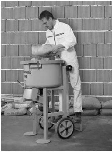
Figure 3. Filling Mixing Tub
