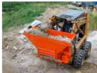
Level Hog Crusher and start recycle process.
