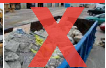
Stop paying to have recyclable debris removed from the job site.
