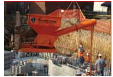
Extended auger tube saves several feet of boom extension
