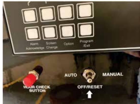
**Figure 32. Auto/Manual Switch (Off/Reset Position)**
