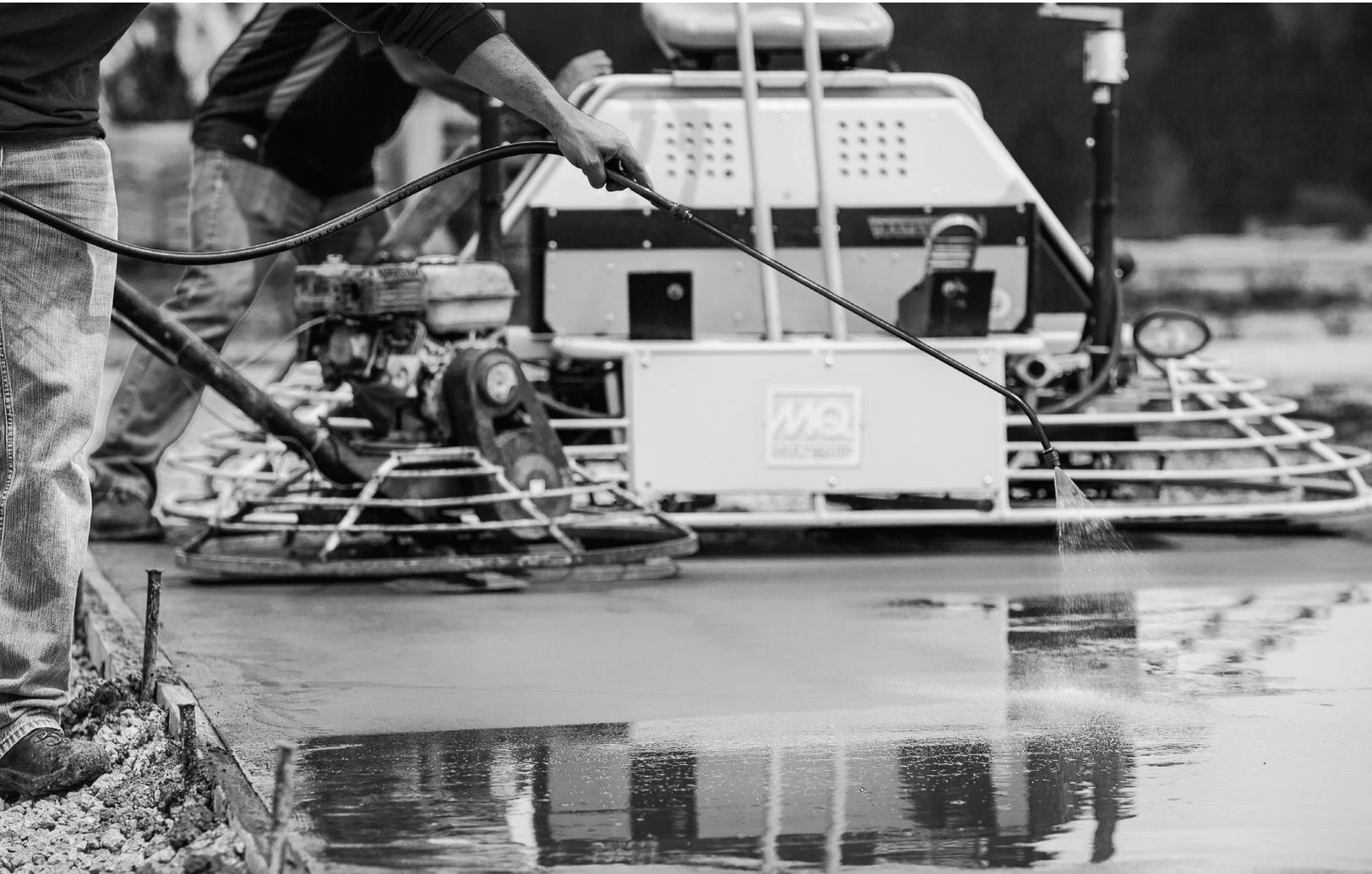
***SlabArmor™ Closer is a spray-on, leave-on condensifier that dustproofs and hardens in a single application with minimal clean-up.***
