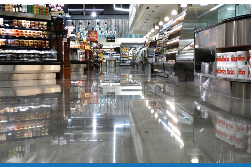
This reactive penetrating product forms an insoluble chemical bond to produce a dense sealed surface, with superior hardness, enhanced gloss and slip resistance.
